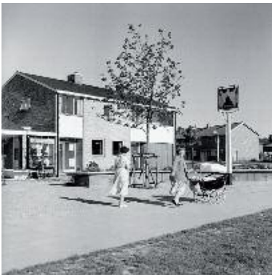
New Town Harlow (UK), 1950s.
